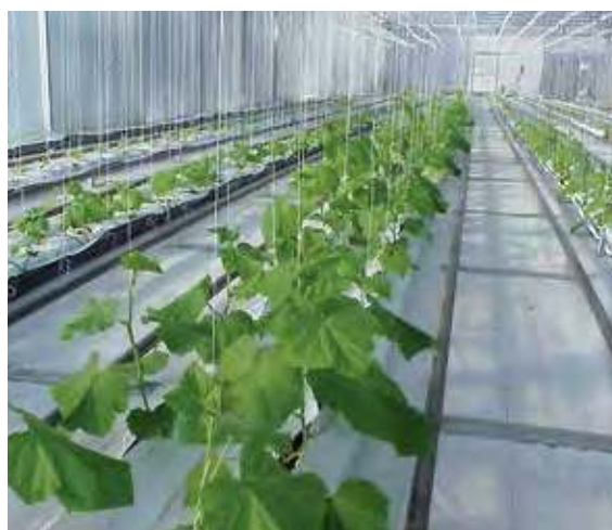
Top and above: Hydronic heating pipes can double as trolley rails to improve efficiency.
