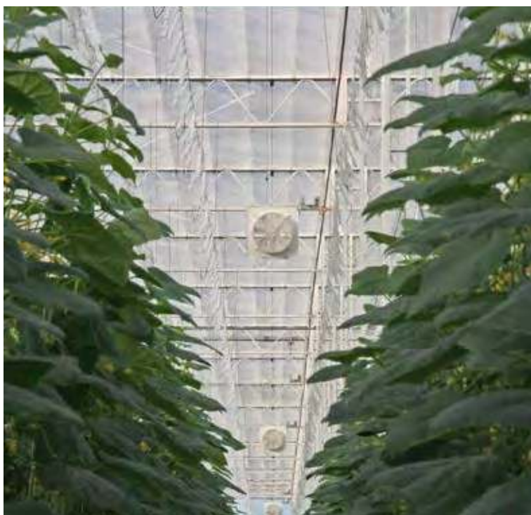
Horizontal Air Flow (HAF) fans are used to circulate air within the greenhouse.
