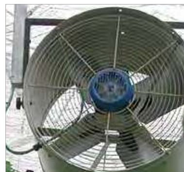
Horizontal Air Flow (HAF) fans are used to circulate air within the greenhouse.
