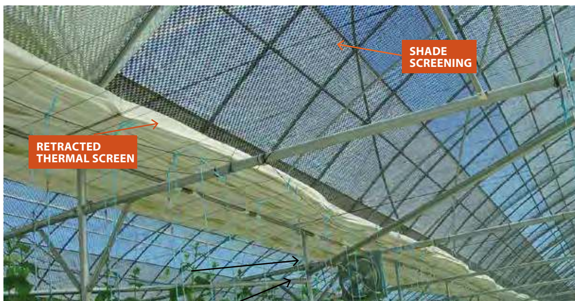
Use of both thermal and shade screens.
