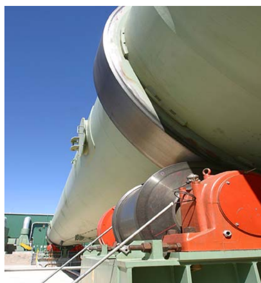
Figure 7. In-vessel composting. (Southern Metropolitan Regional composting facility, Canning Vale, Perth)
